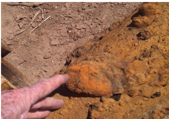
Figure 8. A water well pump encrusted with iron rust tubercles. Photo by G. Hix.
