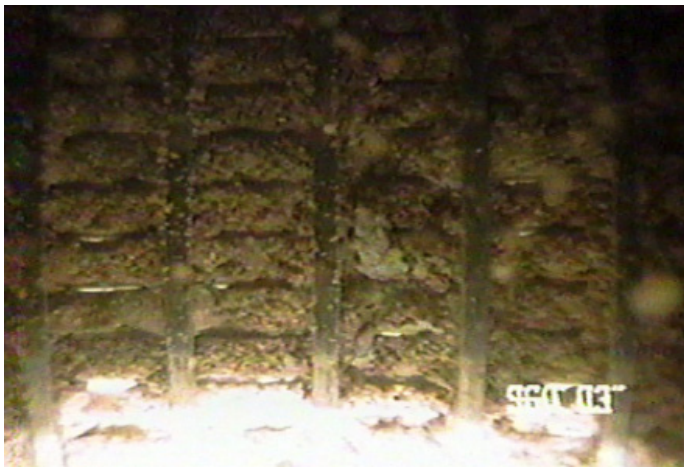
Figure 7. Wire wrapped well screen plugged with slime and mineral deposits. Photo by G. Hix.
