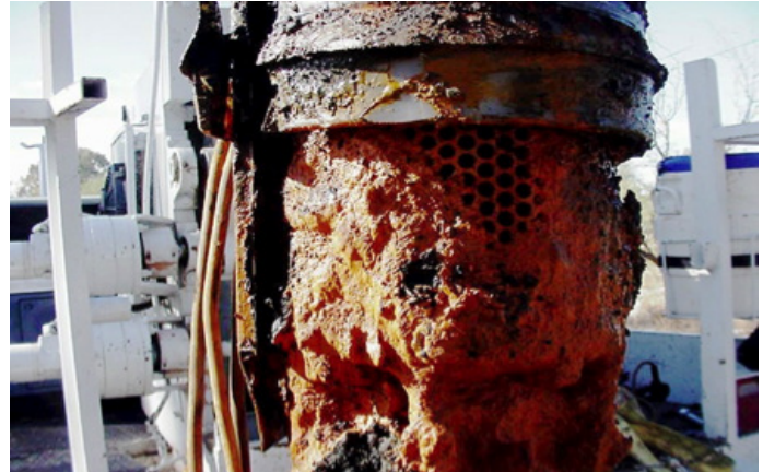
Figure 6. A well pump intake screen covered with red slime and iron rust formed by bacteria living inside a pumping well. Photo by G. Hix.
