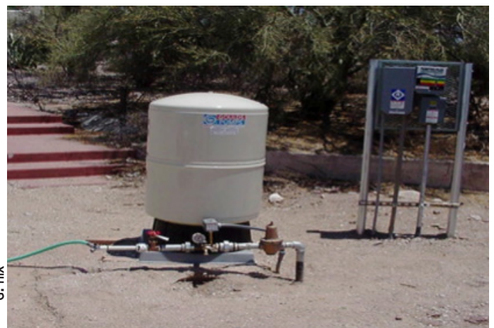
Figure 1. Typical Domestic Well System with Pressure Tank
